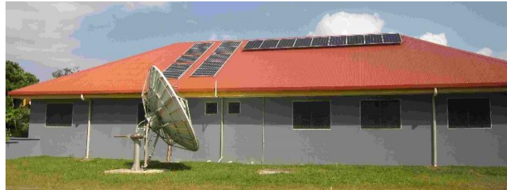
Figure 3.1: PV-powered Satellite Communications, National Bank of Vanuatu, Aneityum
