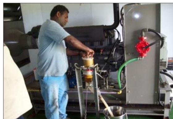
Figure 3.5 40kW Biofuel Generator, Port Olry Source: Port Olry case study (PPA, 2010)
