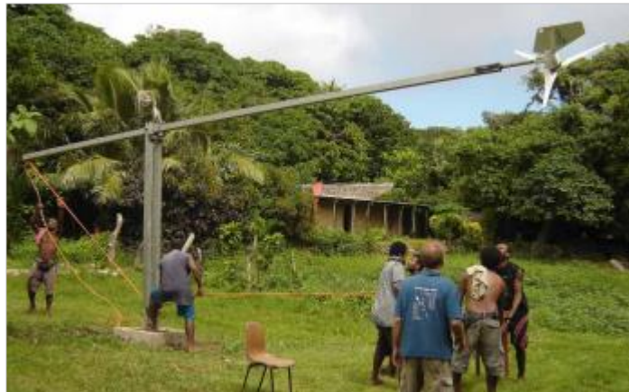
Figure 3.8: EU-VANREPA wind system installation, Futuna, Tafea Source: UNDP, 2012
