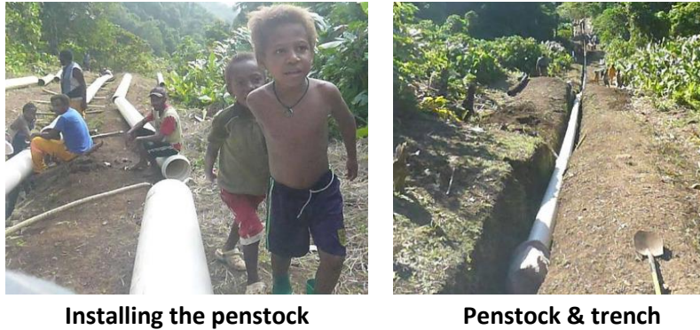
Installing the penstock Penstock & trench Figure 3.7: Construction of Talise hydro Project Source APACE; http://www.apace.uts.edu.au/docpublish/Talise.html
